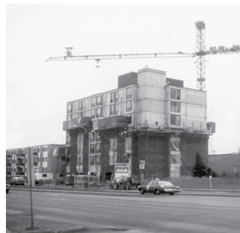
▲ Good Samaritan Place under construction in 1982
